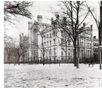
Located on Washington Square, the 1835 main building of the University of the City of New York (now known as NYU)—designed by Town, Davis & Dakin to recall the Gothic spirit of Oxford and Cambridge—was an early “mixed-use” structure containing classrooms, studios, laboratories, and apartments for faculty members.
